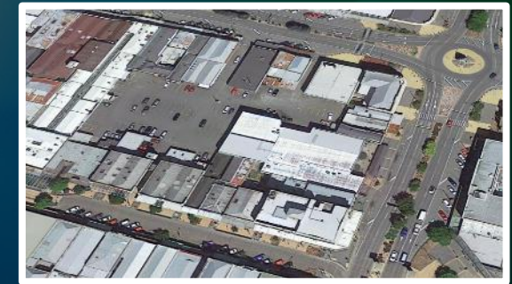
LAND & BUILDING INVERCARGILL, NEW ZEALAND*
