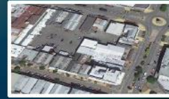
LAND & BUILDING INVERCARGILL, NEW ZEALAND*
